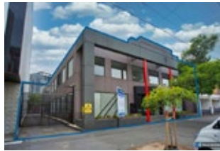
A Commercial Building
