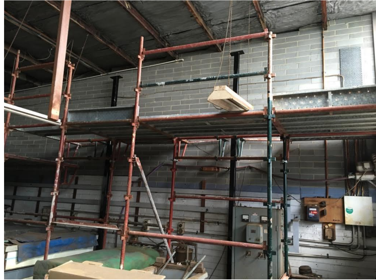
Fire Separation Works
